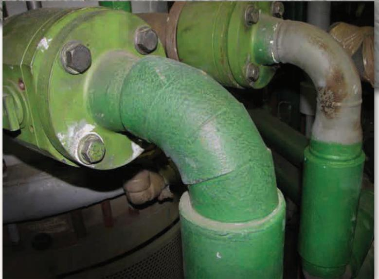
Thin insulation avoids damage during pipe installation without cladding
