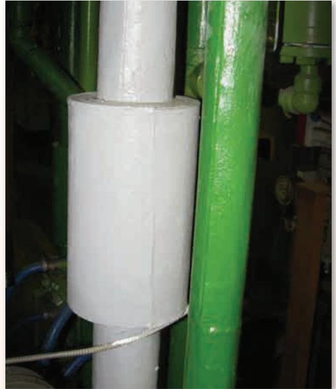
LEFT: Operators work continuously in the web of pipes, often coming into contact with them. Aerogel insulation reduced the touch temperature to safe levels, dramatically reducing the risk of injuries.
